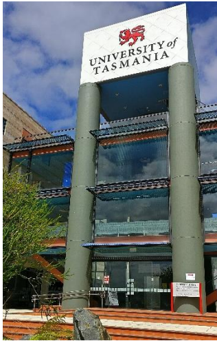
Centenary Building, Sandy Bay Campus
